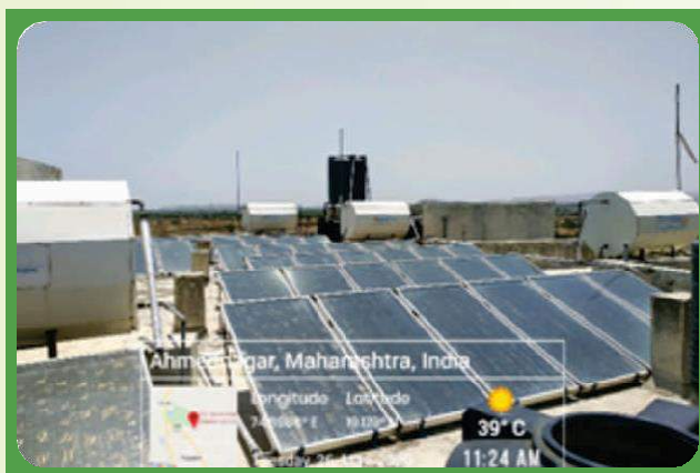
Figure 7 : ETC and FPC solar water heating system
