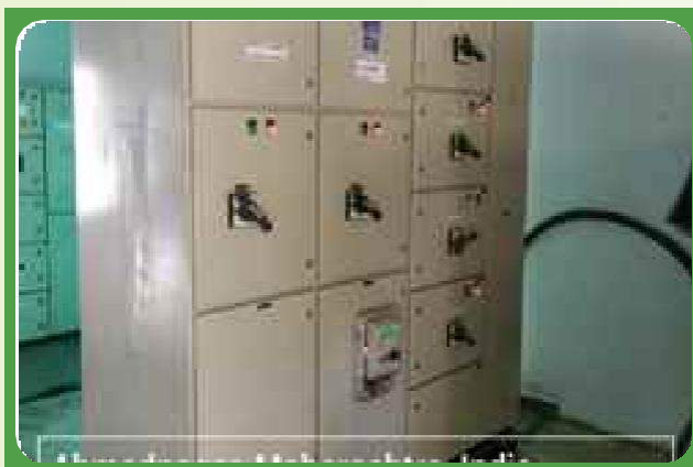
Figure 4 : Meter and inverter panels
