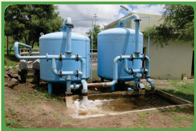
Figure 16 : STP filters and air compressor
