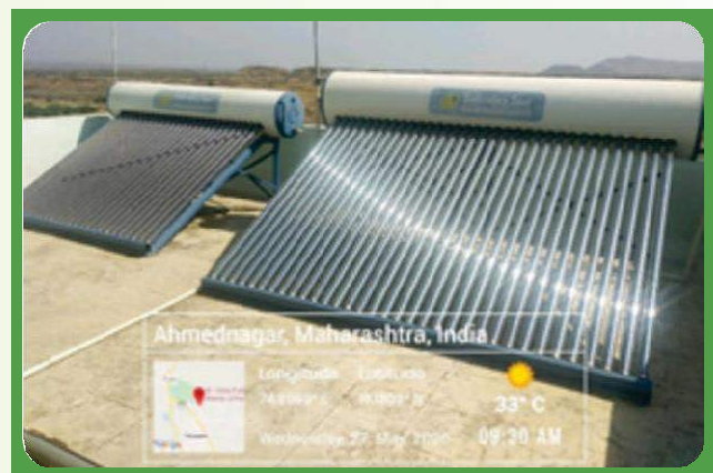
Figure 7 : ETC and FPC solar water heating system
