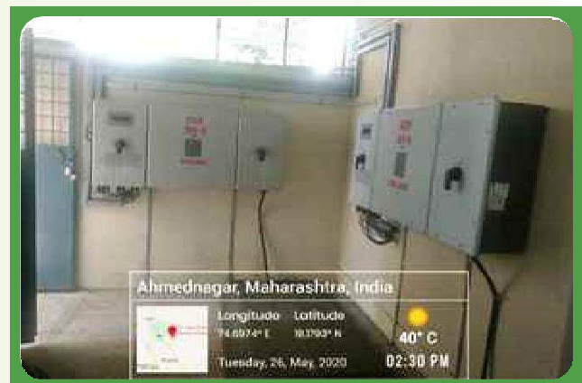
Figure 4 : Meter and inverter panels
